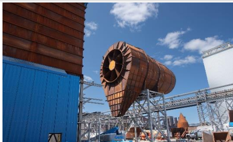
Axial Cyclone installation on Baghouse
