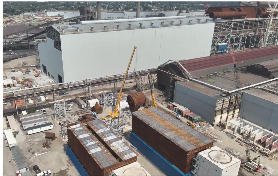
Axial Cyclone installation on Baghouse
