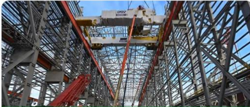
Essential to the EAF process, one of our two 570 ton Danieli cranes has been successfully installed.
