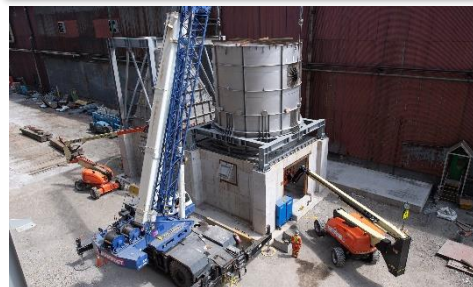
Quench tower assembly is underway
