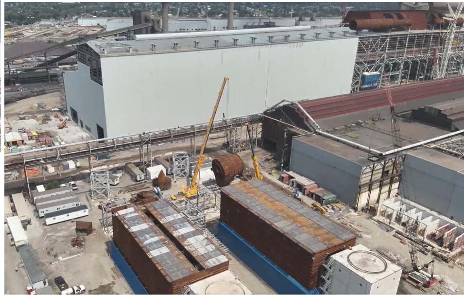
Axial Cyclone installation on Baghouse
